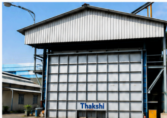
HEAT TREATMENT SHED
