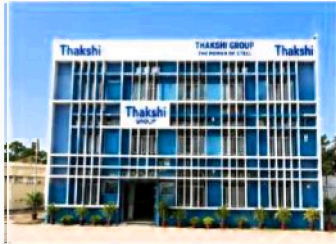
MAIN OFFICE BUILDING
