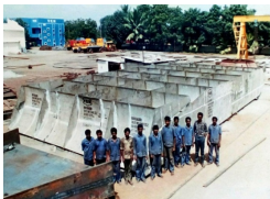
SS GUIDE VANE assembled and fabricated by M/s.VKN INDUSTRIES.
