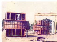
TRAIL ASSEMBLY OF SPIRAL CASING fabricated by M/s.VKN INDUSTRIES for CHANDRAPUR PROJECT.
