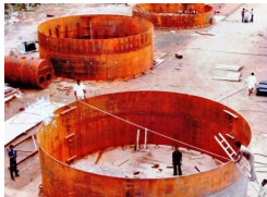
Trail assembly SILOS for CHINA BOILER under a weight of 136 TON fabricated by M/S. VKN INDUSTRIES.
